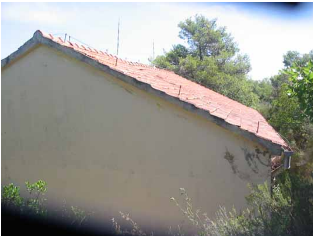
Photo nr.4. View on the south side of the roof and the west wall
